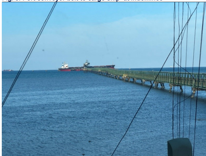
Fig. 8: Port conveyor belt to cargo ship at Indominco
